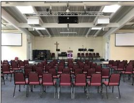
A Trilite lighting bar was installed for the platformfacing LED display and performance LED lighting. The above picture also shows the dual motorised projection screens and Electrovoice ZX speaker system for effective amplification from full-range Worship music amplification to speech. Floor boxes provide discreet but highly flexible connectivity within the platform for musicians.
